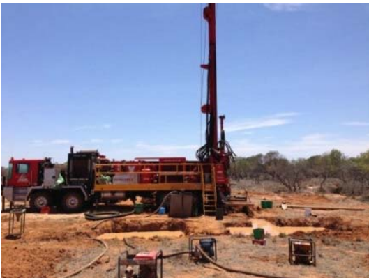
Figure 8: Installing water production bores at Carnavon. Credit: DAFWA
