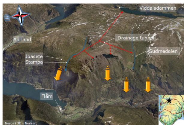
Figure 1: Study area (aerial photography draped over topographic model courtesy of www.norgei3d.no ) indicating areas with known previous rockslides and creeping movements (orange arrows) of both massive rock (fjord) and loose debris (valley) partly driven by pore water delivered by the Stampa and Gudmedalen catchments. Red lines indicate the potential water drainage tunnel system.
